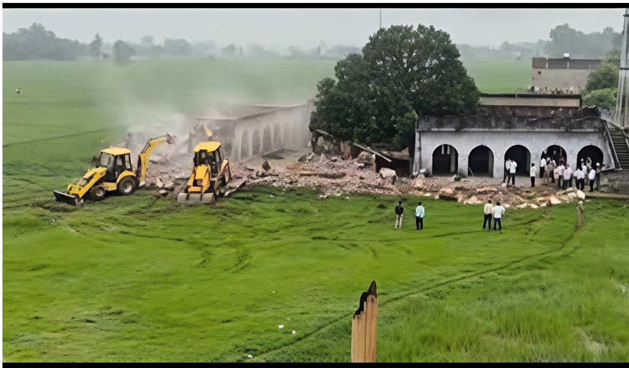
Authorities demolish a 59-year-old madrasa in Siddharthnagar, Uttar Pradesh.
